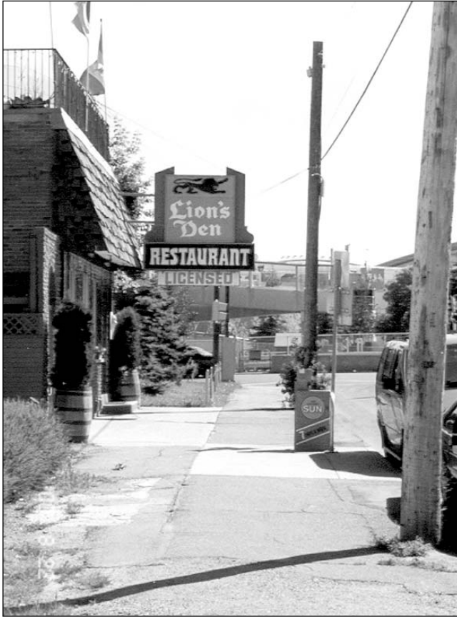
There are places in the Beltline with broken curbs and sidewalks, unattractive utilities, missing boulevards and substandard public amenities and services. These give the appearance of neglect, deter investment and contribute to social deterioration.
