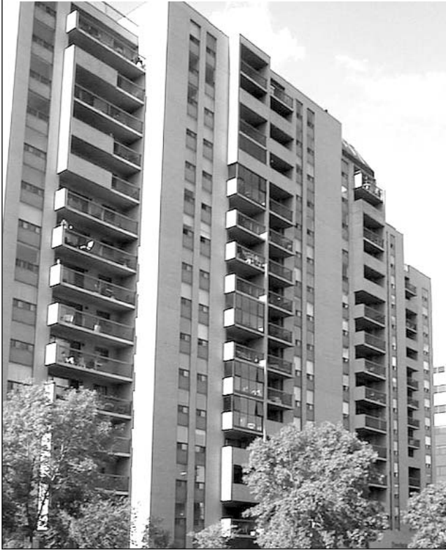
A typical 1980s residential high-rise located along 14th Avenue W.
