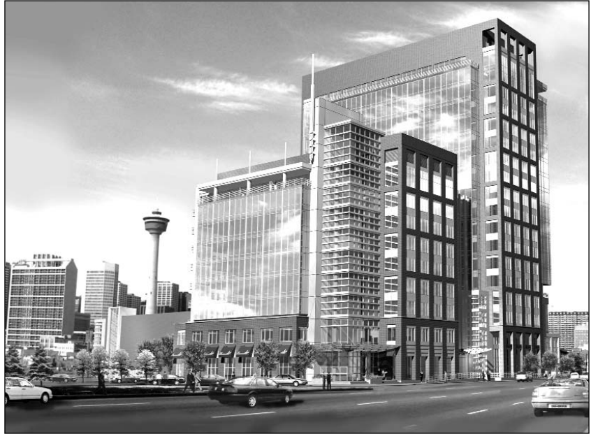
Stampede Station will transform the Macleod Trail corridor as Calgary's major gateway in and out of the Downtown core.
