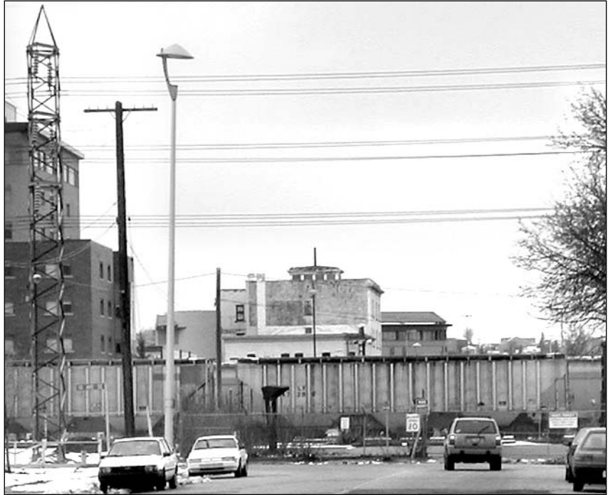
Despite Olympic upgrades, 4th Street E fails to connect the Stampede Grounds to 9th and 6th Avenues in the Downtown. Doing so would alleviate peak use traffic jams and maximize development opportunities in both Victoria and East Village.
