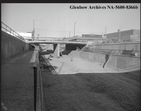
8th Street Underpass
