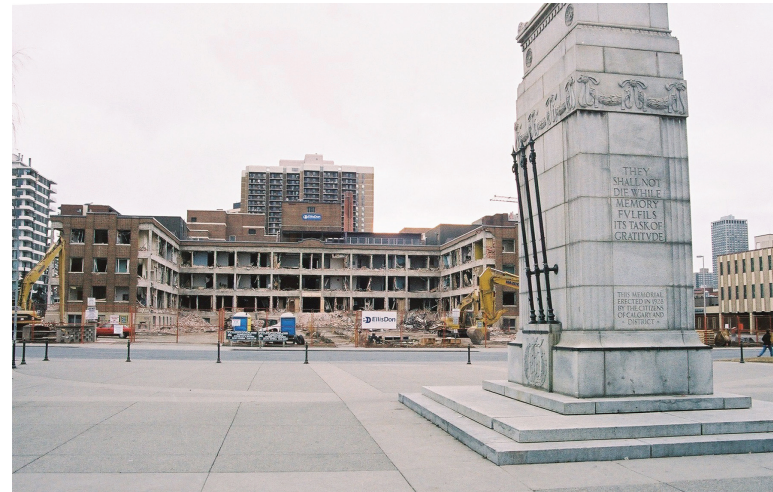
demolition of Colonel Belcher hospital (1919), Calgary, 2007
