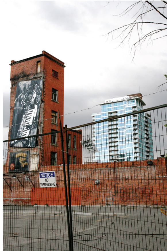
pre-demolition of the Underwood Block Calgary, 2007
